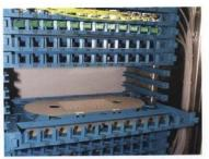
Splice and distribution modules can be inserted in and pulled out freely for operations.
